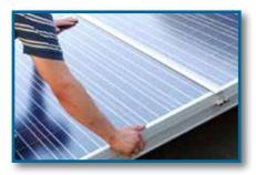
Modules are inserted between parallel horizontal rails. Just place the panel into the top rail, let it slide down and the job is done!
